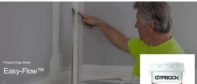
Gyprock Easy-Flow is lightweight all-purpose jointing compound specially developed for mechanical application, with excellent tape adhesion, trowelling and feathering properties.
