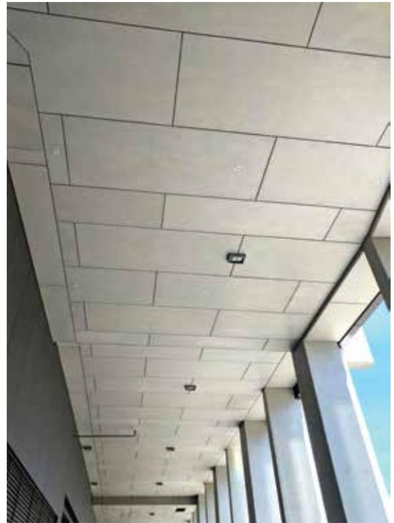
**FIGURE 2.02** 9mm Barestone™ ExpressWall Top Hats
