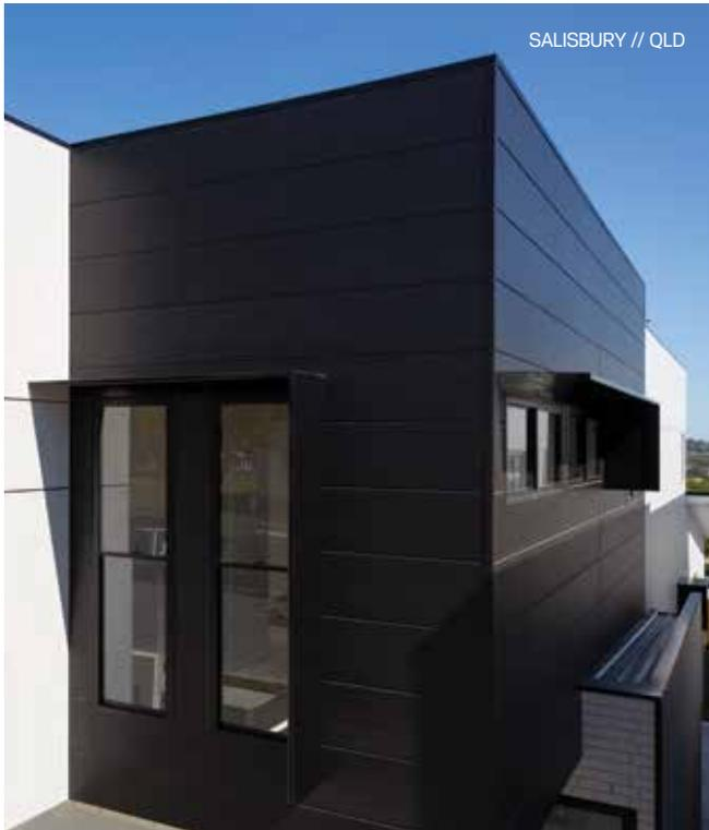
The 300mm wide Cemintel Aspect Cladding® panel displays a single and visible 16mm wide groove, providing easy coverage for an attractive façade.
