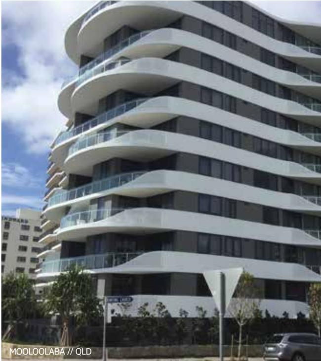
Cemintel Commercial RendaLine® is a complete external cladding system that incorporates all the advantages of lightweight construction with a flush-jointed, texture coat finish.
